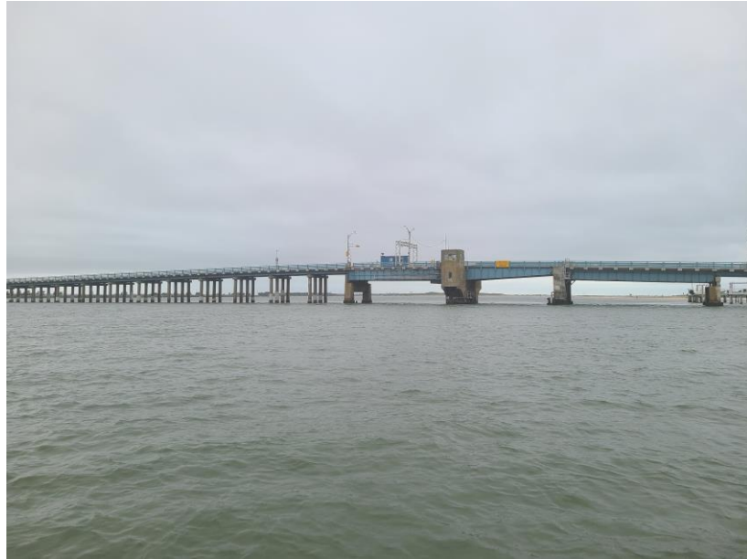
Figure 2. Corsons Inlet Bridge with closed bascule (8/20/2025)
